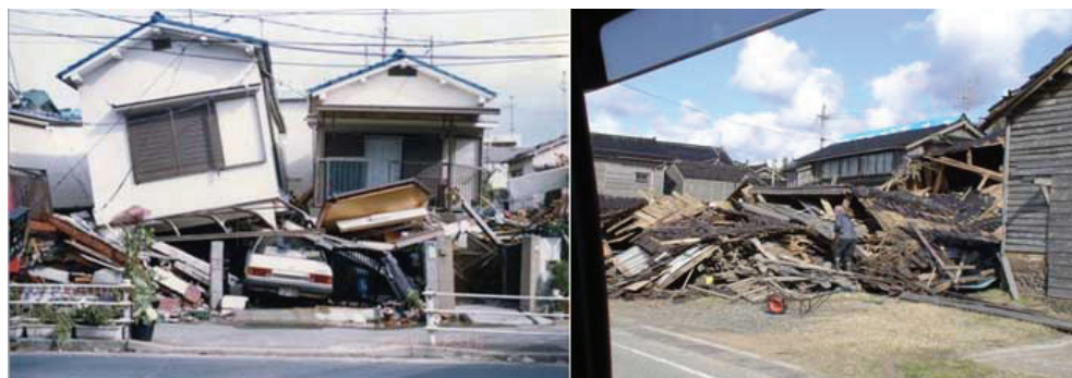
Fig. 1. Collapsed Japanese wooden houses in Kobe (1995, the left figure) and Noto (2007, the right figure) earthquakes
